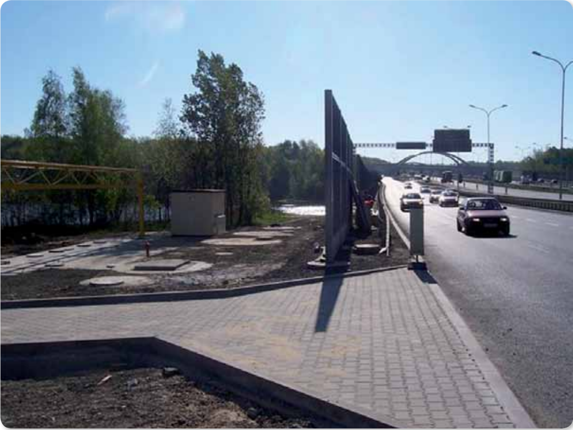
Katowice Sewerage System dry well pumping station with solids separation system ETS
