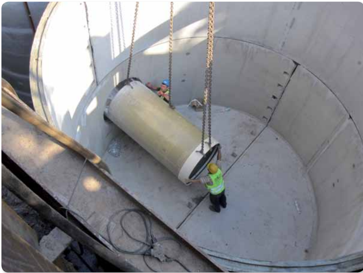
Construction and reconstruction of storm water channels, Gdynia settling tanks, separators
