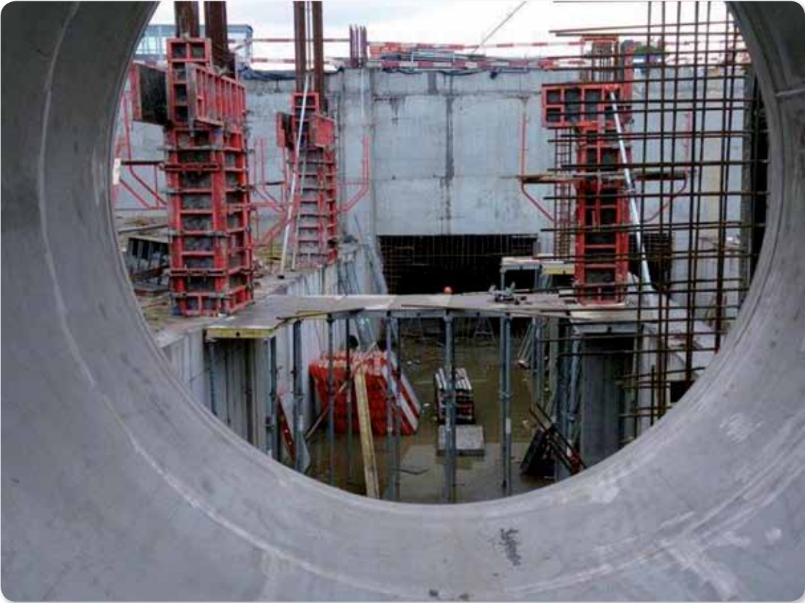
Reconstruction of the water junction, Gdansk pumping station EPS
