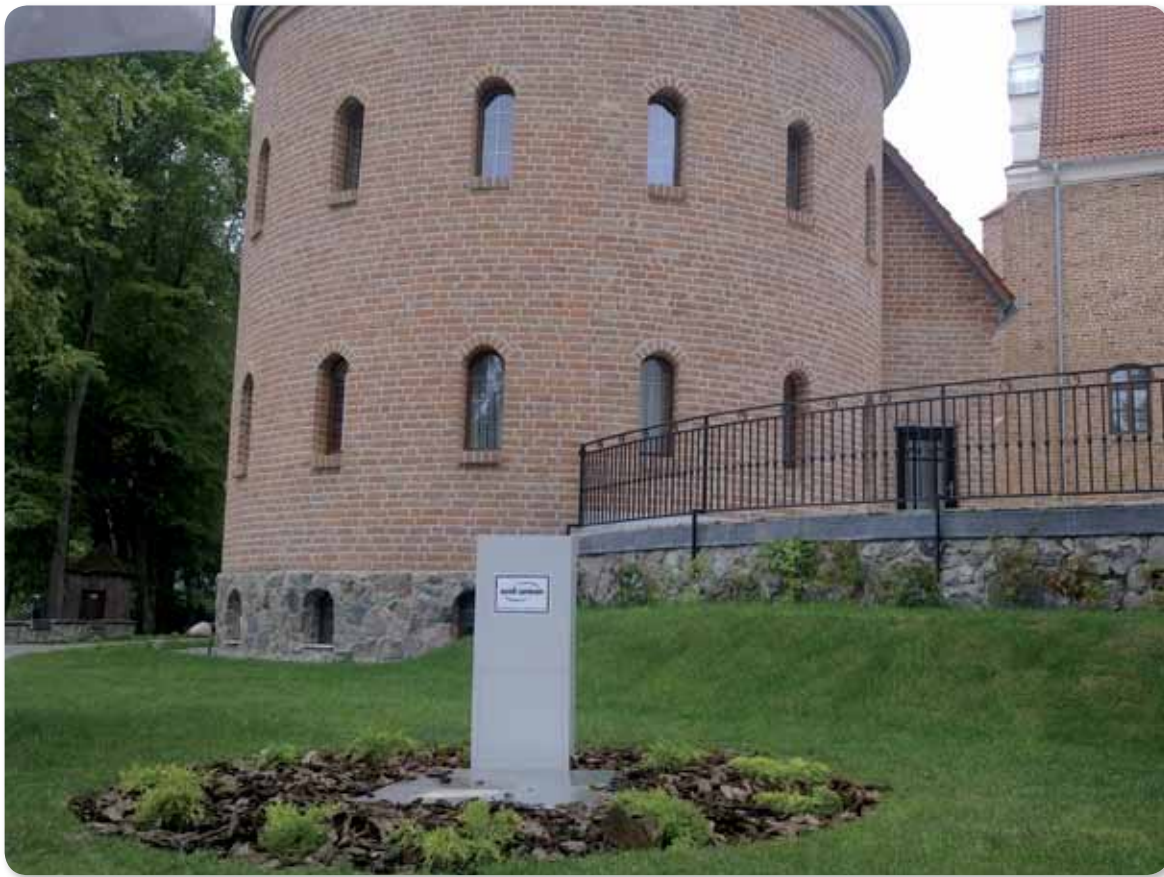
Hotel, Gizycko pumping station EPS
