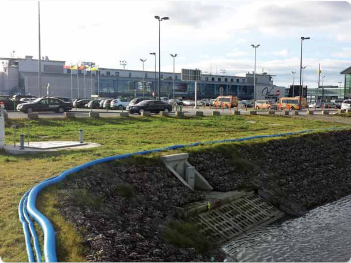
Gdansk Lech Walesa Airport pumping stations EPS, separators, EU chambers, settling tanks
